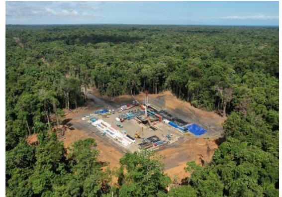
RH Petrogas' Riam-1 drilling site
